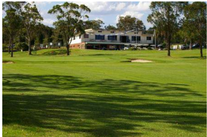
The old Club House prior to renovations. 1970 - 2009
